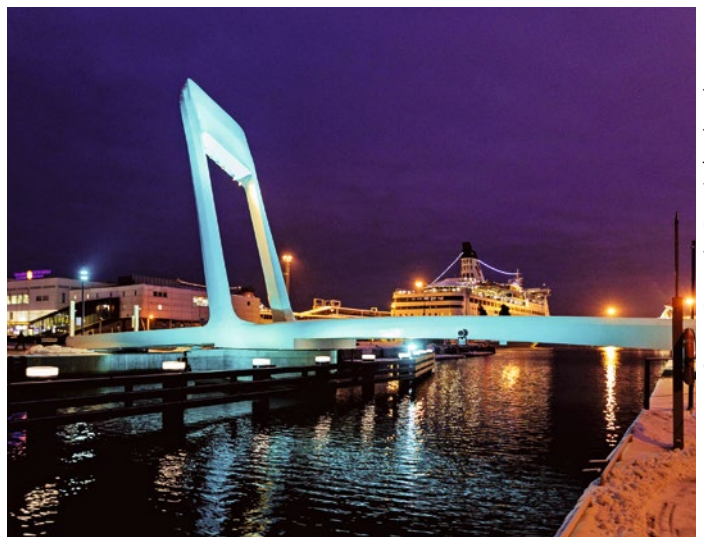
A new pedestrian bridge in the Port of Tallinn
